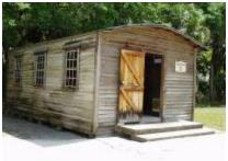
The Small Machine Shop (1905) was responsible for manufacturing specialized tools, kitchen items, and performing clock and watch repairs. It was a modest onestory building with horizontal wood siding and a cypress shingle roof, later replaced by tin. In its history, it experienced only minor alterations, including a small metal addition to its southwest corner, and modification of the entry doorway. <sup>54</sup>
